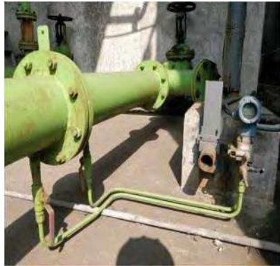
Water meter @inlet line
