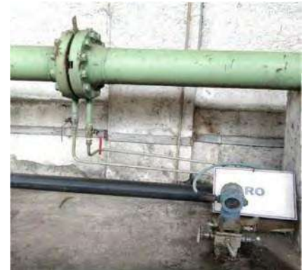
Water meter @reuse line
